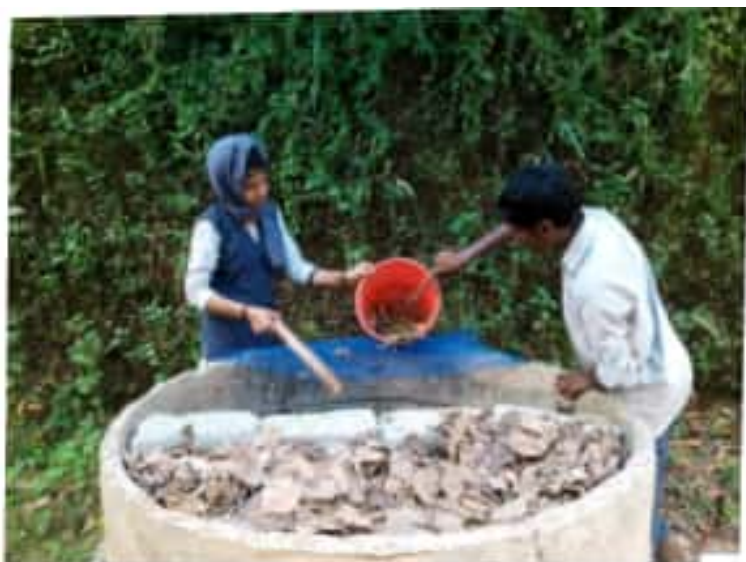
Our Ring Composting System to deal with Bio Waste
